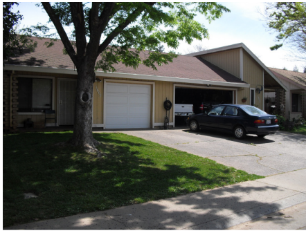
Corner View of the Duplex
