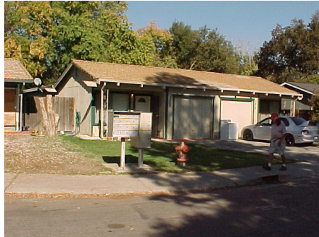
Duplex on the Right Side
