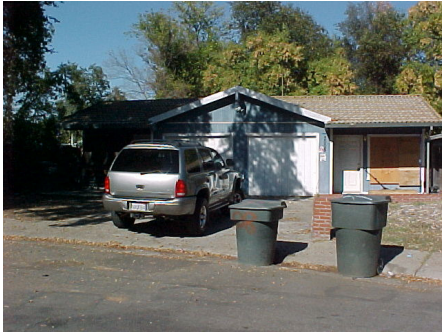
Front View of the Duplex
