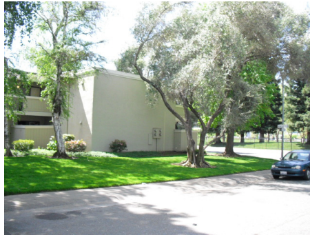
View across the street
