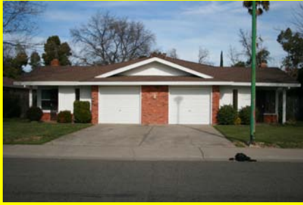
Front View of the Duplex
